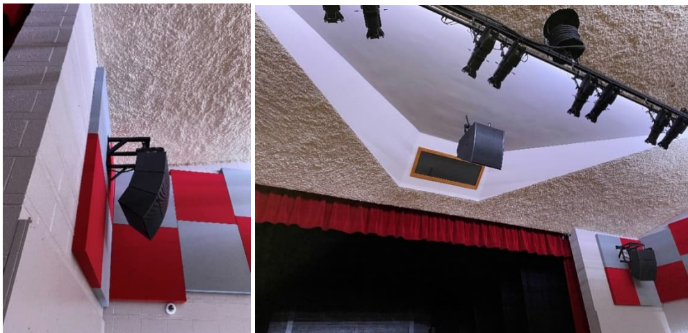
Figure 22 - More installation photos of the loudspeakers and front corner panels
